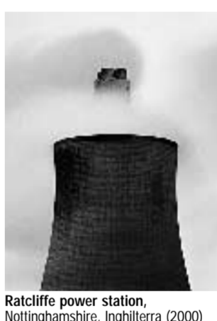
Ratcliffe power station, Nottinghamshire, Inghilterra (2000)
